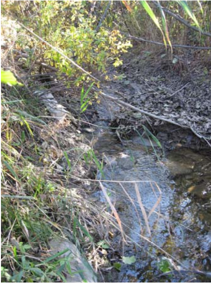
Station 9 : Ponceau route 243
